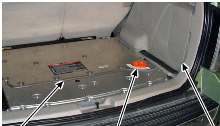
High-Voltage Battery Pack
